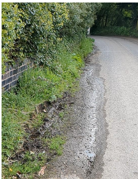
Image above shows water bubbling up through road outside Primrose Cottage, Dark lane, Sinton Green.
