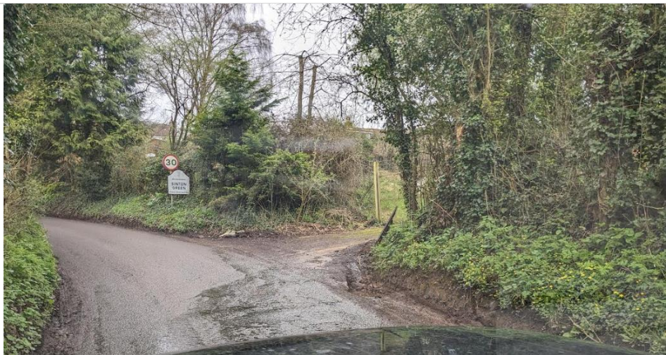
Image above shows water coming out of the Severn Trent facility and shows the eroded road surface.
